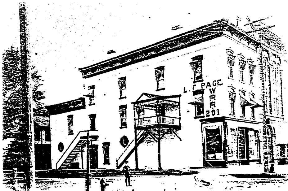
Fig. 8. Page's Store, East Michigan Avenue, Marshall, Michigan, c. 1895.
